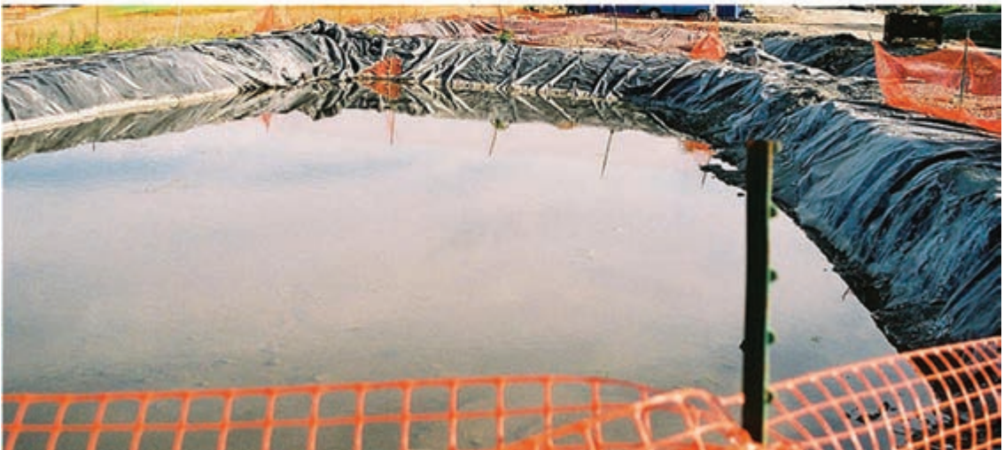
Silpaulin water storage tank
