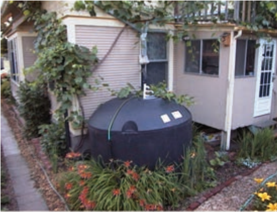
Rain water storage tank
